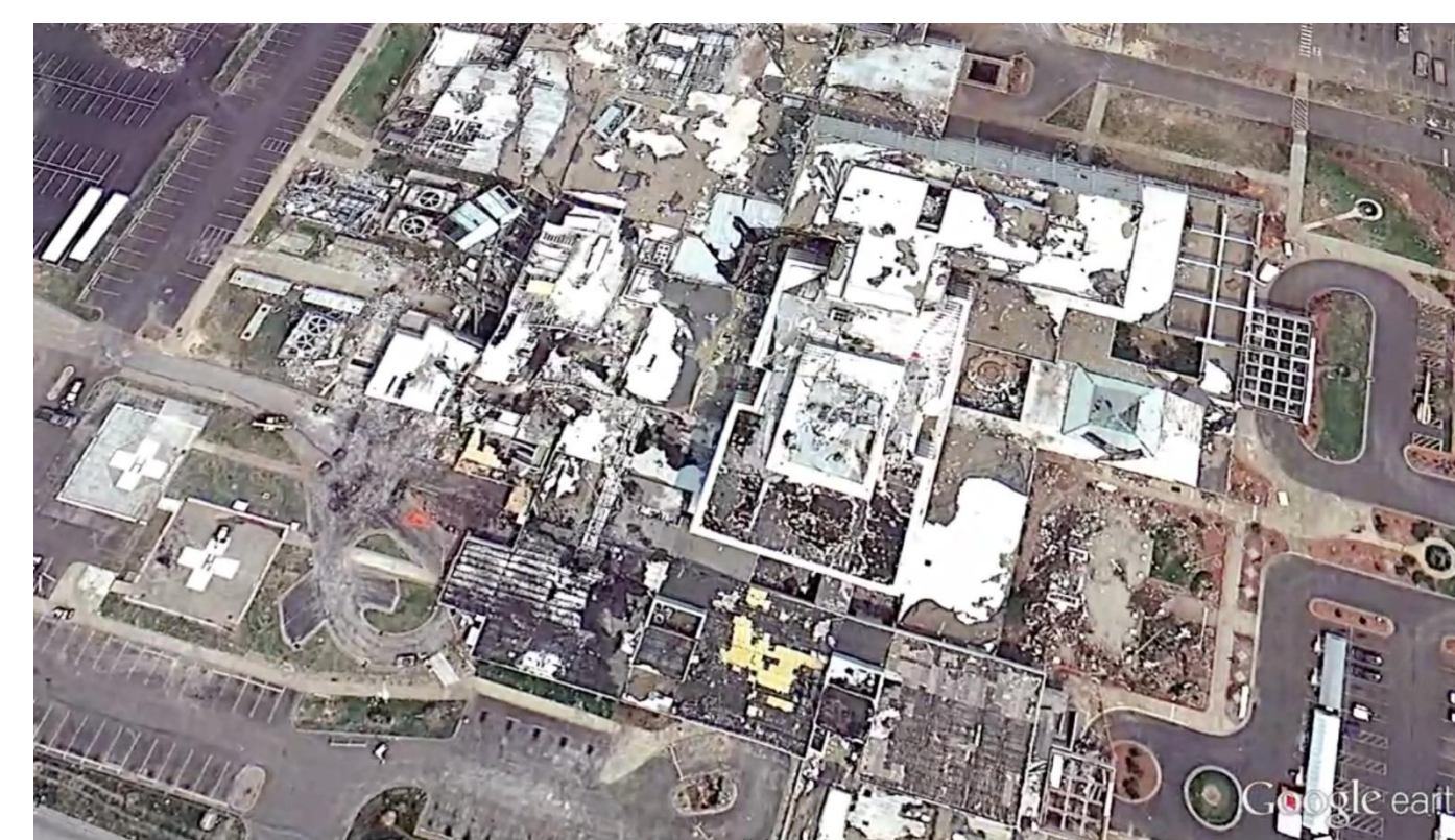
Figure 1: Mercy Hospital in Joplin MO, After tornado impact in 2011
